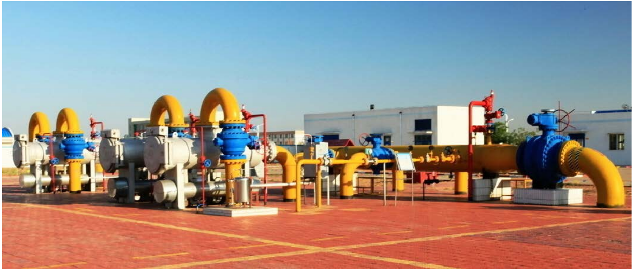
Fig. 4. YODO's Ball Valve installing on pipeline
