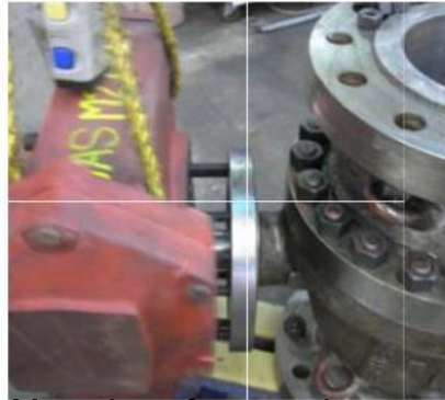
Fig.16. Mounting of gear units on valve.
