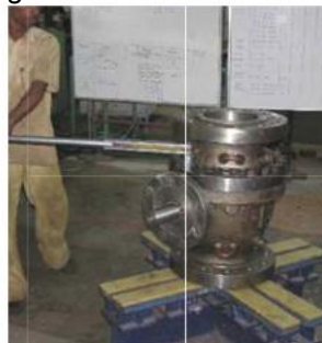
Fig.15. Valve interface flange tightened using a torque wrench
